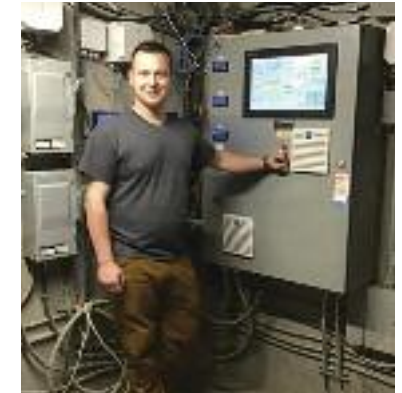
Ryan Weddel, the third generation in the family running Newmarket Pre-cast, uses this computer to set the ingredient levels in a given batch of concrete. Different concrete products require different mixtures. Photo by Conrad Boyce
