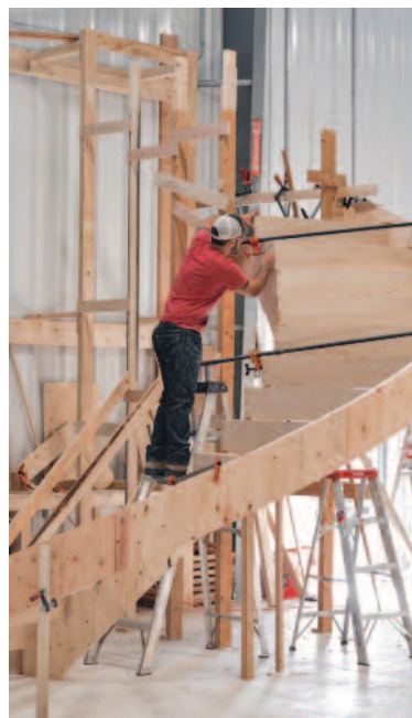
A craftsman at Deluxe Stair and Railing assembles a custom curved staircase.
